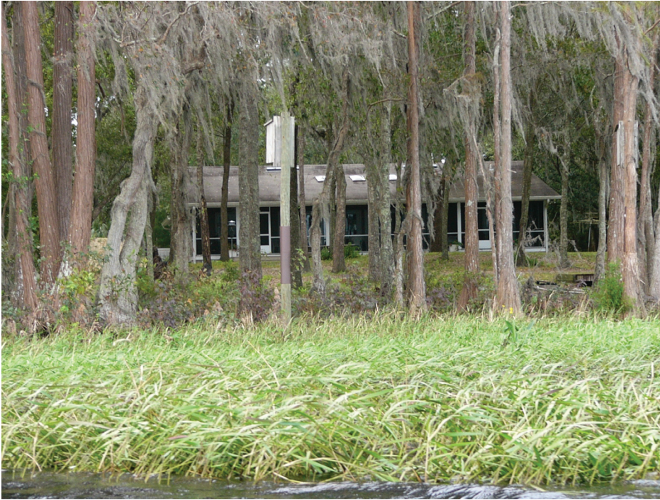
Example of a healthy shoreline. The house is set back from the water with the natural buffer zone intact.
